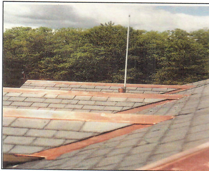
This is a flat cap installed on the ridge of a house.
